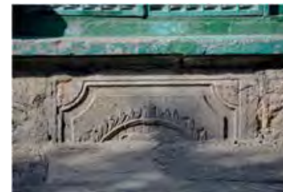
Figure20. The external stone plinths of the building consist of five pieces of carved stone, part of which is hidden in the covering of the current passage (Archive of Tehran City Beautification Organization)
