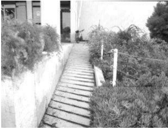
Picture 1. ramp and its suitable slope
