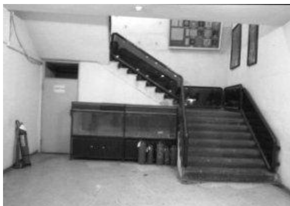
Picture 3. elevator to access the second floor is not installed
