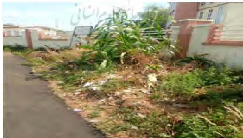
Fig. 8: View of littered surroundings with poor landscape drainage system
