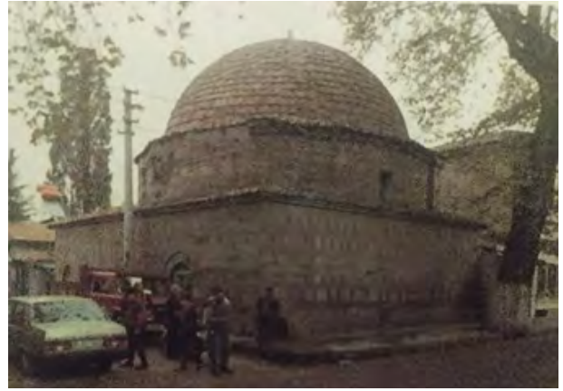
Figure. 8: A view of Haji Uzbek Mosque in Iznik city (Blair, 2002:155).
