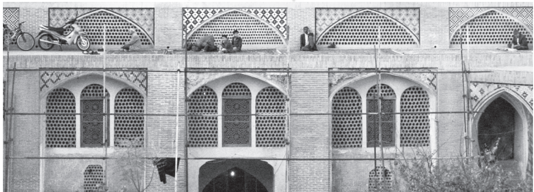
▲ Figure 2. Stone latticework windows in Aqa-Bozorg mosque-school.
