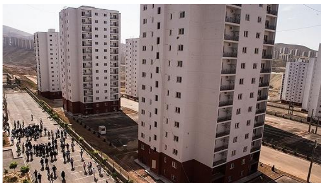
▲ Picture 7. Phase 5 – location of Mehr Housing project in phase 5
