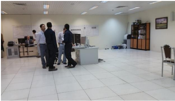
Fig. 1. Control room of Zagros gas power plant
