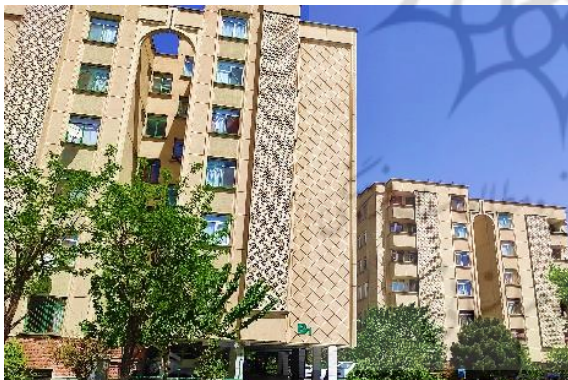
Fig. 3. Sadra residential complex, 2th Sector of 22th District in Tehran
