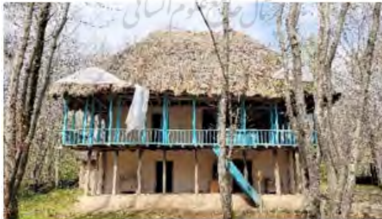
Fig. 7: Using timber and soil in building houses and rice stems for the roof covering in the Gilan Plain rural houses (remade model of Mousavi House at Gilan Rural Heritage Museum)
