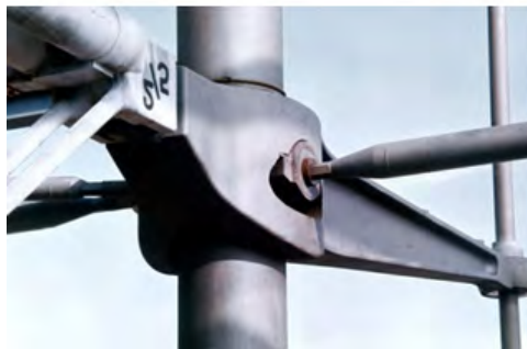
Fig. 11: The type of connections and joints used in the project of Georges Pompidou Center. France. 1977 (Source: Denancé & Berengo Gardin, 2017)
