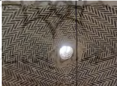
Fig8: Kohfteh Rasteh Brickwork (a style of brickwork) in Colambo source: the authors
