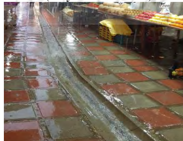
Fig9: Drainage gradient for disposing the surface water of the pathways in Asef Bazaar
