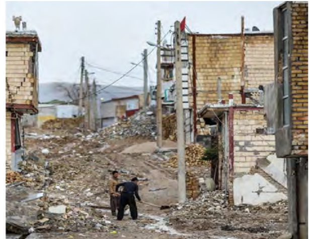
Figure 16. Access Blocked (Source: Authors)
