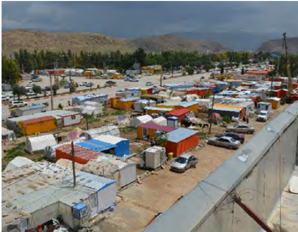
Figure 15. Temporary accommodation on the north side (Source: Authors)
