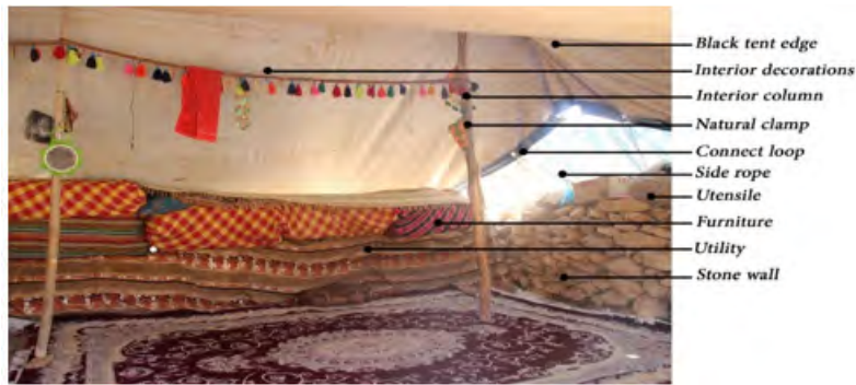
Fig. 11: Interior components of the black tent and its special decorations
