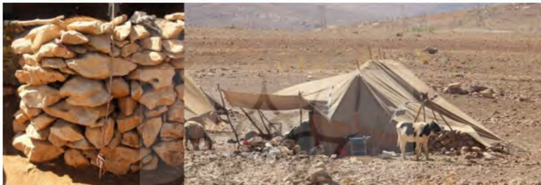
Fig. 19. Arrangement of the stones without mortar.
