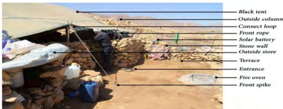
Fig. 12: The elements of a black tent
