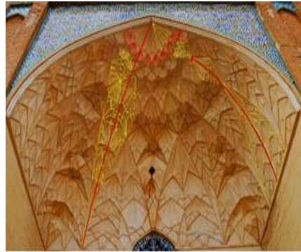
Figure 13. The Aali Qapo entrance to a height of seventeen meters from the buildings of Shah Tahmasb I Safavid with unique decorations and bedding. Continuity, coherence, and rhythm in the levels of connections in organizing the arches covering the entrance, with geometric expansion concentrated to the center. Source: Author.
