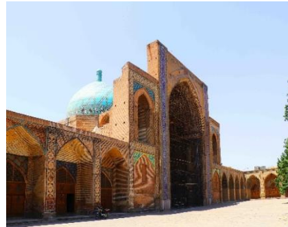
Figure 11. Tiled dome of two shells of Al-Nabi Mosque in the city of Qazvin. Source: Author.
