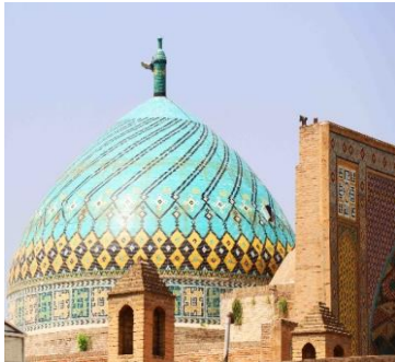
Figure 10. The south porch of the Jameh Mosque of Qazvin with all kinds of plaster and carved tile decorations attached to the mausoleum and an inscription in Kufic script made of gypsum mortar on the stem of the dome. Source: Author.
