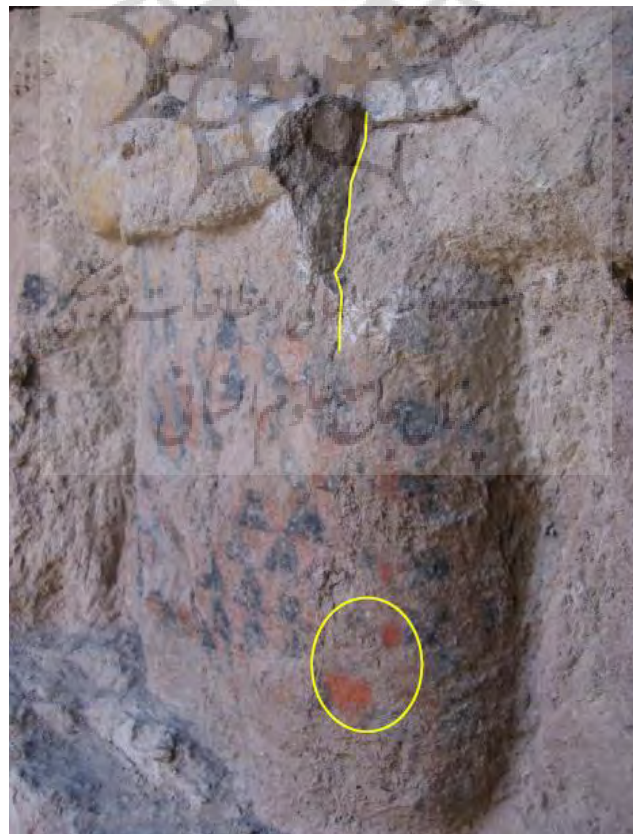
Fig. 10. Fall of left forearm of the relief and continuous crack in hand-wall interface (Author, 2006).
