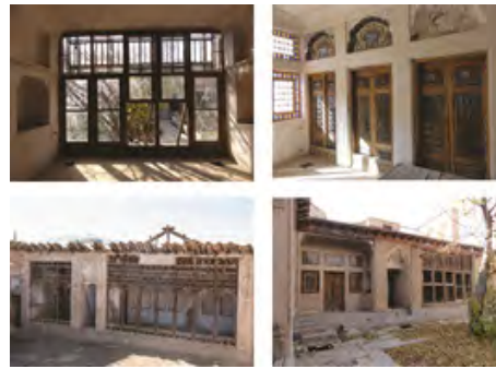
Fig.4: Door, window and Orsis in the building.
