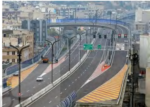
Fig.4: Discontinuity of Sadr elevated highway noise barriers. (Source: Ghorbani, 2013)
