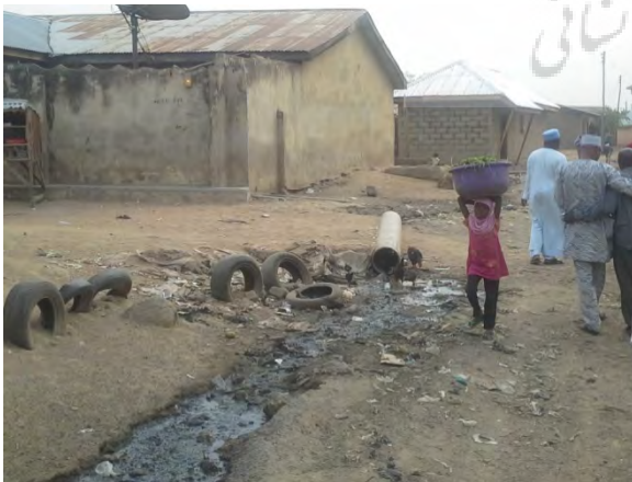
Fig. 2: Unplanned drainage cutting through the road Barkin-Sale area of Niger State, Nigeria (Source: Author's fieldwork, 2013)
