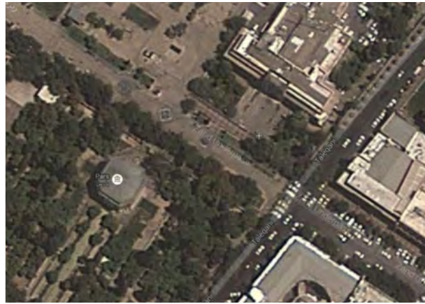
Fig. 5: Aerial photographs from the area and to determine the scope of design and location of shading obstacles (trees) in proportion to the seats. (Source: Wikimapia (2014))
