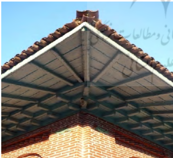
Fig.9: Wooden Beams under the Roofs
