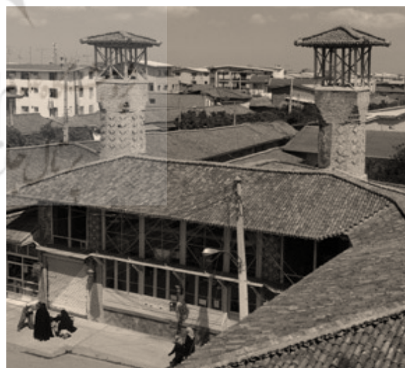
Fig.6: Gable Roofs in Panjshanbe-Bazaar Covered with Tiling
