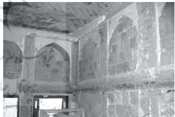
Fig. 10: Discovery of covered Vaults during the layering operation
