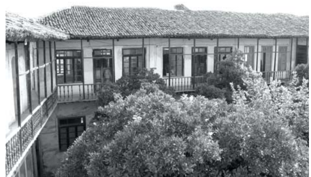
Fig. 6: A view of the northern front of first family courtyard before the restoration operation
