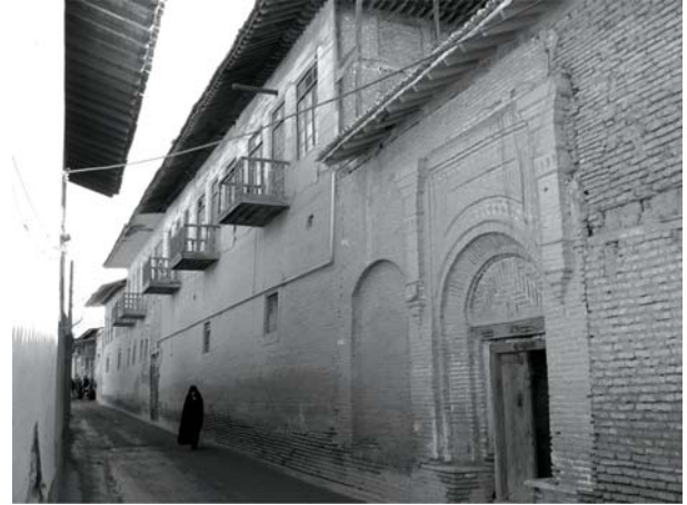
Fig. 5: Main façade of the house from the northern passage before the restoration operation
