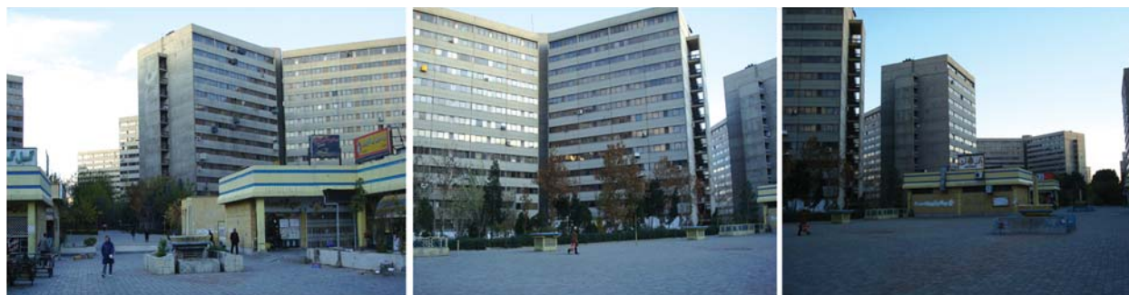
Fig.3,4 &5: Multy-family Housing in Ekbatan
