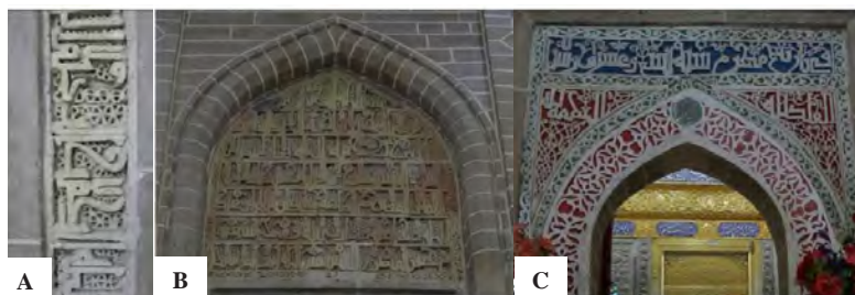
Fig.6. Inscriptions on the entrance to the main dome; (A) Part of the inscription on entablature of the entrance door; (B) Inscription of the ordering authority; (C) Inscription of the construction date
