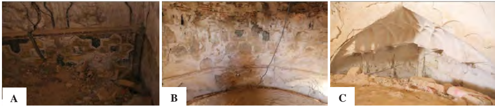
Fig.11. Remaining artifacts between the skull and the chipped dome itself; (A) Colored stuccos between the outer surface of the cap dome and the chipped dome; (B) Transitional phases in building a chipped dome; (C) Remaining artifacts from Mocárabe corners of the dome
