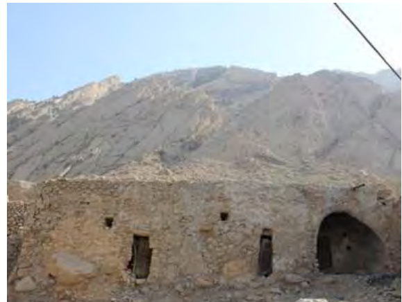
Fig.13. Very small doors and windows facing the mountains and facing the sun in a rectangular plan house in the Dinavars neighborhood. The Langar mountain is visible in the image background.
