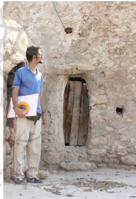
Fig.15. The entrance to a house where most of the points mentioned are evident; Being small, use three slices of palm wood and lintel stone protruding from the wall
