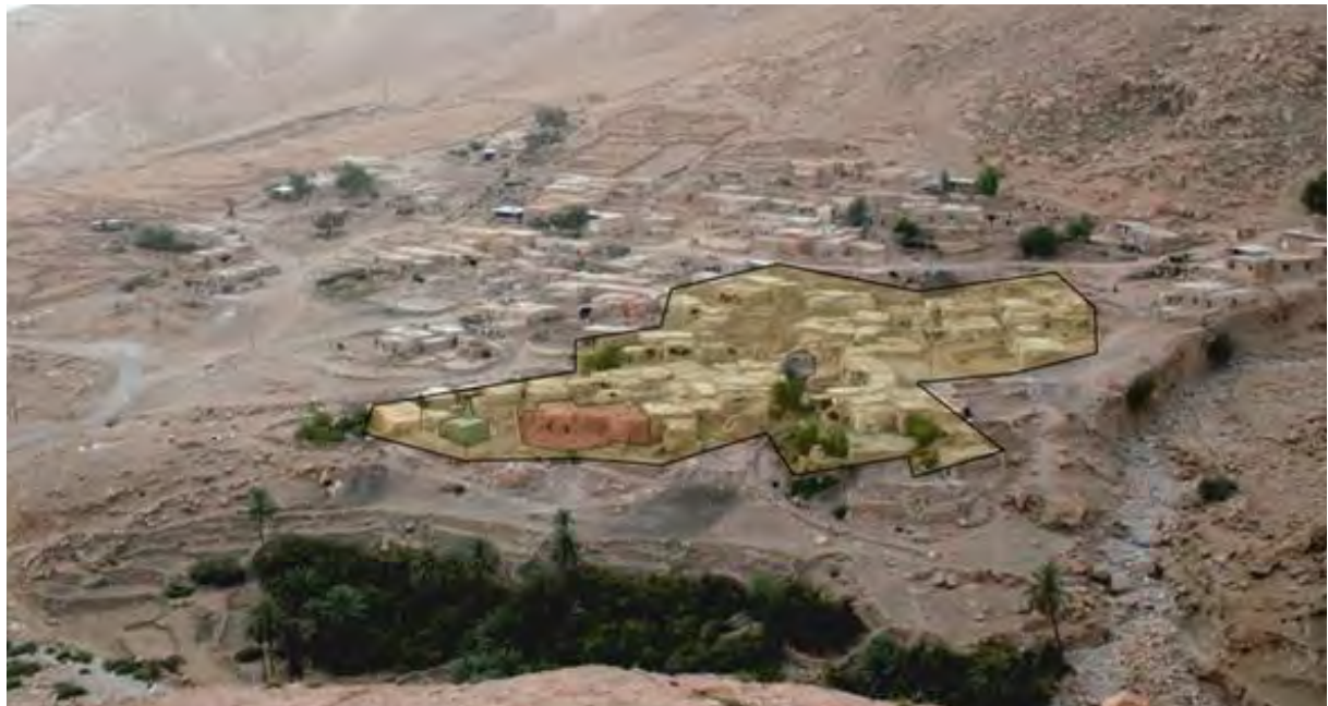
Fig.4. Overview of the village from the southeast; The Dinavarha district is marked in yellow, the Ghadamgah in green, the castle in blue and the complex presented in the pictures in red.
