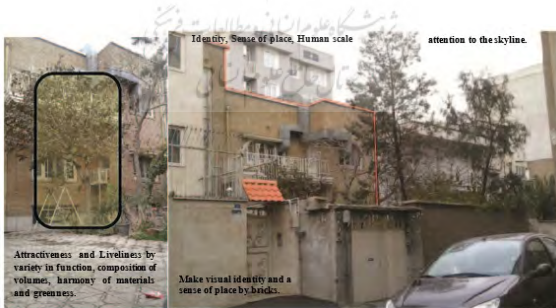
Fig. 13: Indexes of Identity, Sense of Place, and Human scale in the façade of located in the Monirieh region.
