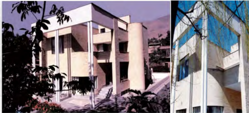
Fig. 9: The facade of a residential building in the Zaferanieh region, Tehran. (Source: Saremi, 2012)
