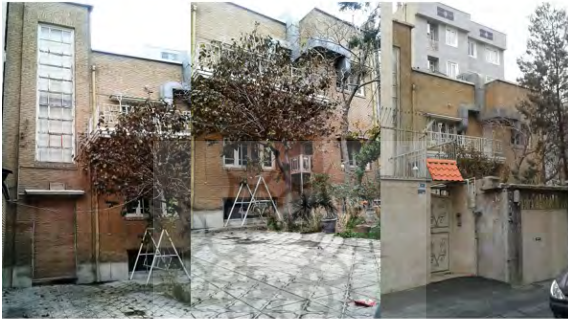
Fig. 6: The facade of a residential building in the Moniriyeh region, Tehran.
