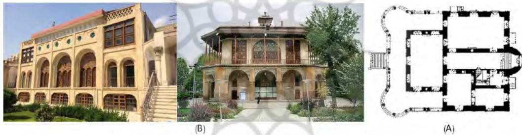
Fig.8: Azizieh or Malijek Mansion. (A) The plan of Malijek Palace. (Source: Saadati Khamseh, 2016) (B) The facade of Malijek Mansion. (Source: Zakarzadeh, 2008).
