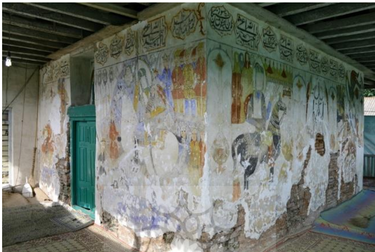
Fig. 2. Building Construction of Agha Seyed Ali Buq'a-Motealegh Mahaleh-Lahijan
