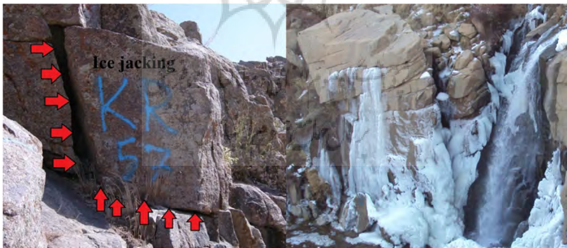
Fig. 7: A view of blocks detaching due to ice jacking action
