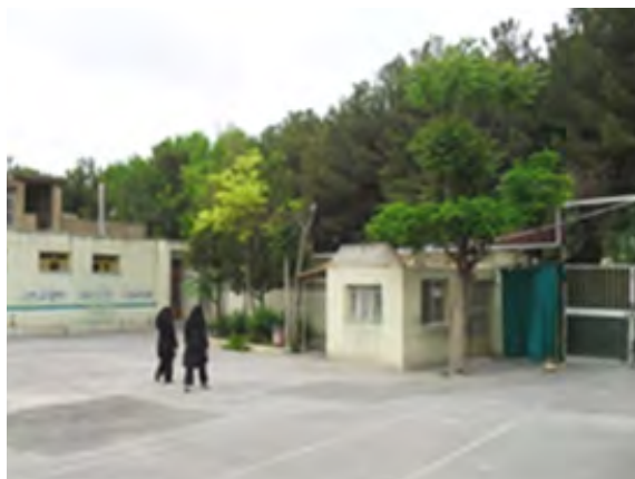
Fig. 13. Poor quality and improper design of outdoor space in Niayesh high school
