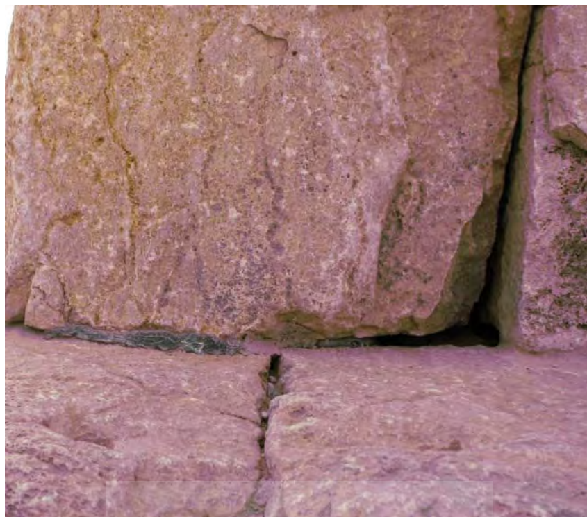
Fig. 2 Achaemenid Used the Lead as Mortars for Connecting Rock Fragments. Place: Tomb of Minor Cyrus, Bozpar
