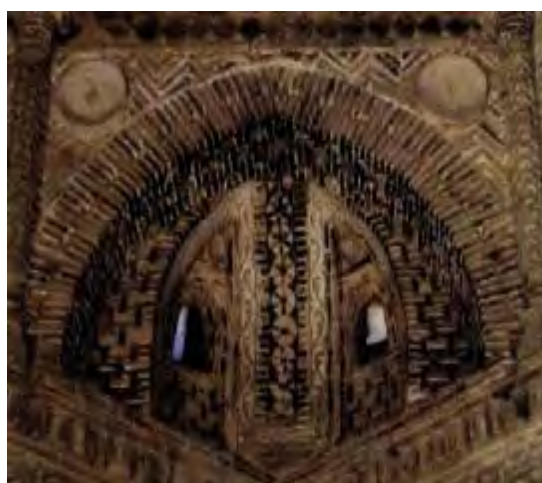
Fig. 6 Interior view, squinch supporting the dome (Ibid)
