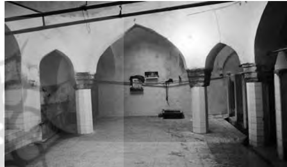
Picture 5 Small hot-house, Haj kazem bath – In Qajar period, the change of the function of water reservoir made the dimensions of the hot-houses smaller. (Photograph by author)
