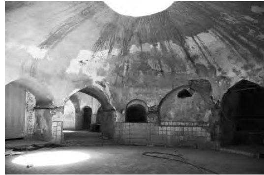
Picture 4 The large hot-house, Sheykh Bahaei bath. (Photograph by author)
