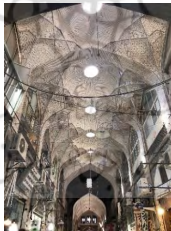
Fig 9. View of ceiling orifices
