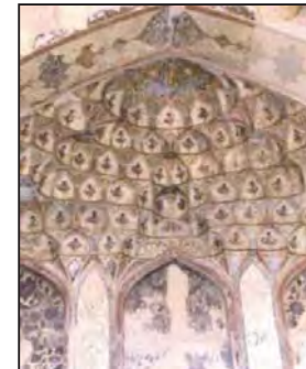
Fig. 14 Overview of the ornamentation of the southern side of the room
