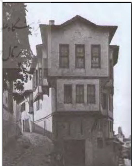
Fig.11. Forming consoles to exterior volume. Source: Goodwin, 2009: 605.
