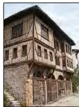
.Fig. 4.Wooden framin gand filler materials Source: Midilisari, 2011: 785
