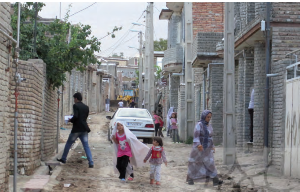
pic2: Partnership is a necessary issue in order to unite the government and the public in the modernization measures and to compensate for delayed justice and it's realization. Uromieh deteriorated fabric, photo: Abolfath Sepanloo, 2013.
