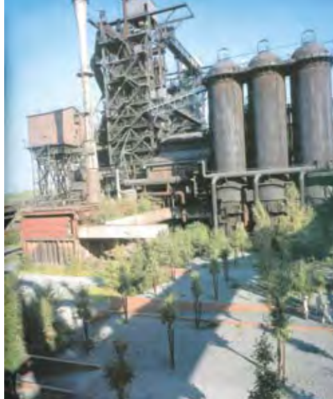
Pic 4, 5. Re – interpreted with a new syntax, peter latz interlaced existing fragments into a new "landscape". Source: Weilacher: 2009.
