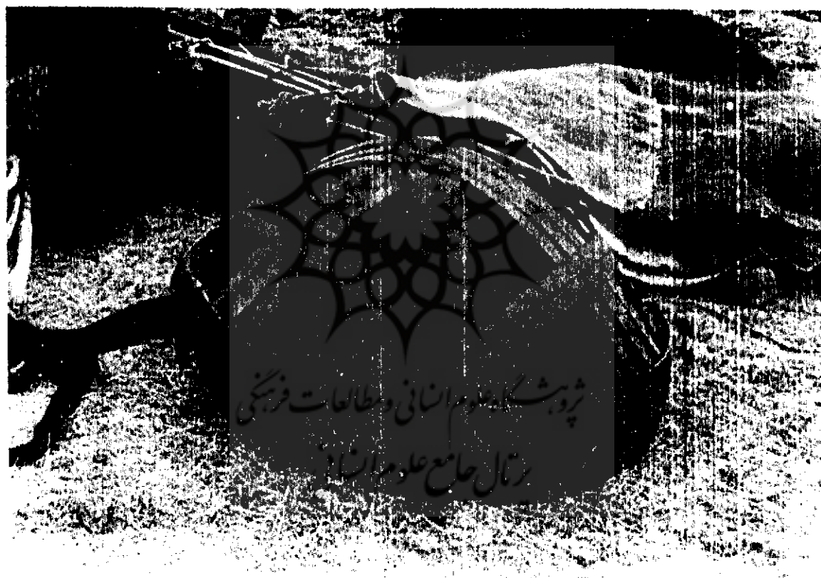
Roof ring, with struts beyond. The great circle laths are paired.
