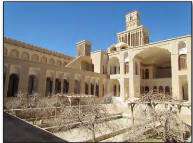
Fig. 3. A wind-catcher in Yazd, Iran. It is both a symbol of Iranian architecture enjoying innate visual identity (vaults and arcs) and a structure similar to other Iranian architectural monuments. Source: author's archive.
