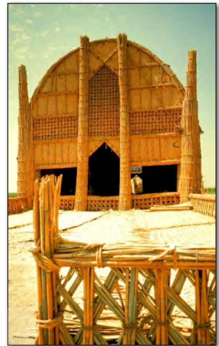
Fig. 6. A reed-made house in Shadegan lagoon, Khouzeestan. Source: Mojtahedzade, 2013: 60-65.
