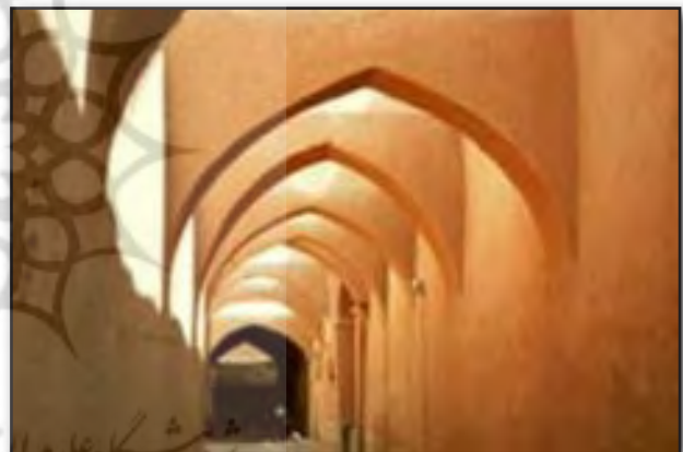
Fig. 4. In this picture, several visual features are present of which the negative space is outstanding. The view of vaults and the depth created as well as mud-straw mixture, as locally available material, are among identity-creating features of this structure. Source: author's archive.
