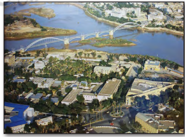
Fig. 5. white Bridge and former literature faculty (triangular) as signs in Ahvaz. Source: Khuzestan governor, 2013.
