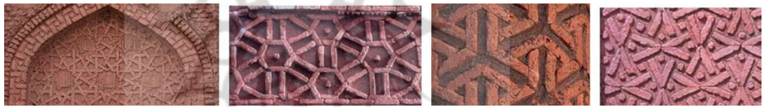
▲ Fig 6.Tower of Kharqaqin Qazvin, 12-point, 6-point, abstract 6-point, and8-point geometrical patterns
