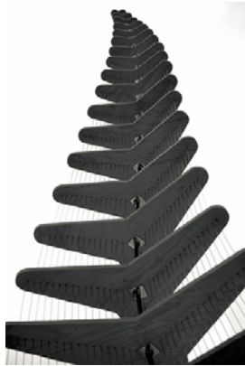
▲ Pic 1. Draw-strut frame system (Frei Otto); sources: author.
