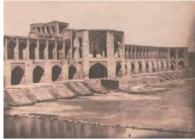
Fig.5. The structure above Khajoo bridge, an addition by Sadr Esfahani (Hoeltzer, 1976: 120)
