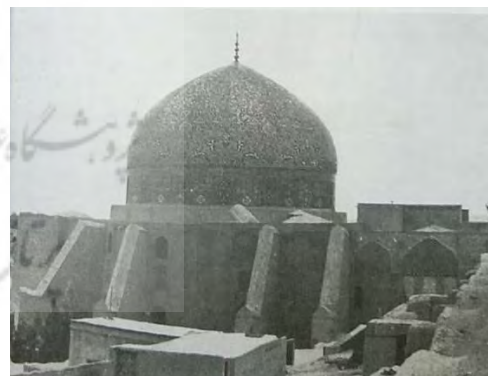
Fig.15. Addition of buttresses to Sheikh Irfollah mosque (Zander, 2017)
