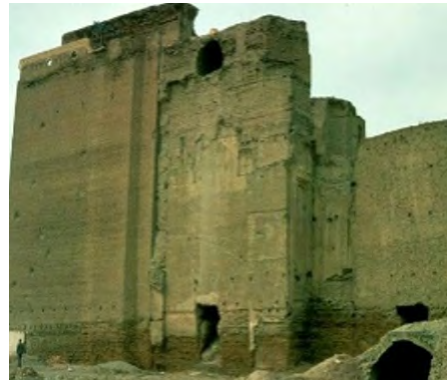
Fig. 4: Exterior view of the western wall
