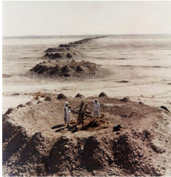
Fig .3: Windlass as a main implement of shaft digging. (Source: Rashedi, 2016 A)
