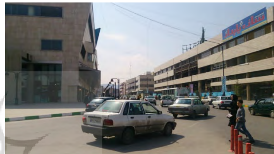
Fig. 5: Square Exterior Chambered, Toos: Building
