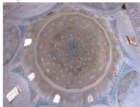
Fig. 14: The central part of the dome
