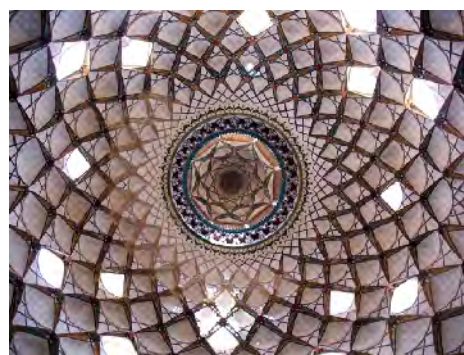
Fig. 18: Openings in the middle of Yazdi-bandi units across the ceiling, Boroujerdi-ha house
