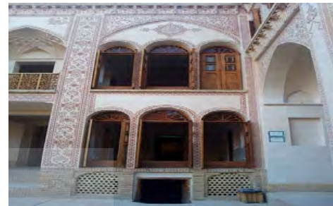
Fig. 2: Shebak in basement and Door-Windows in first and second floor.
