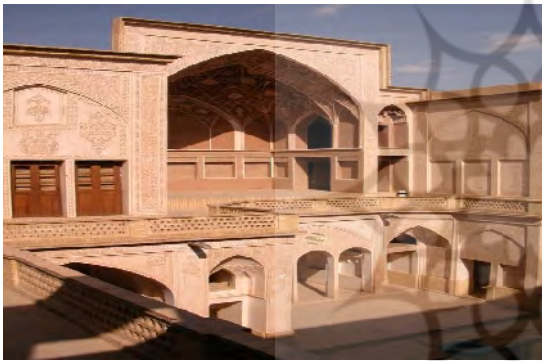
Fig. 8: The building in the second floor is set back to provide better access to the sun. Abasian House, Kashan, Iran.
