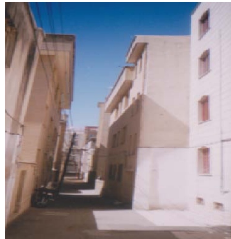
Fig. 4: high density and being surrounded degree in Hasanabad zargande district, region3of Tehran municipality. (Source Authors)
