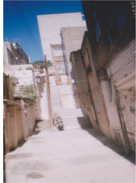
Fig. 6: Non- standard stairs and two much height of eroded houses, not observing technical criteria, on the slope of Gheitarieh hill. (Source Authors)
